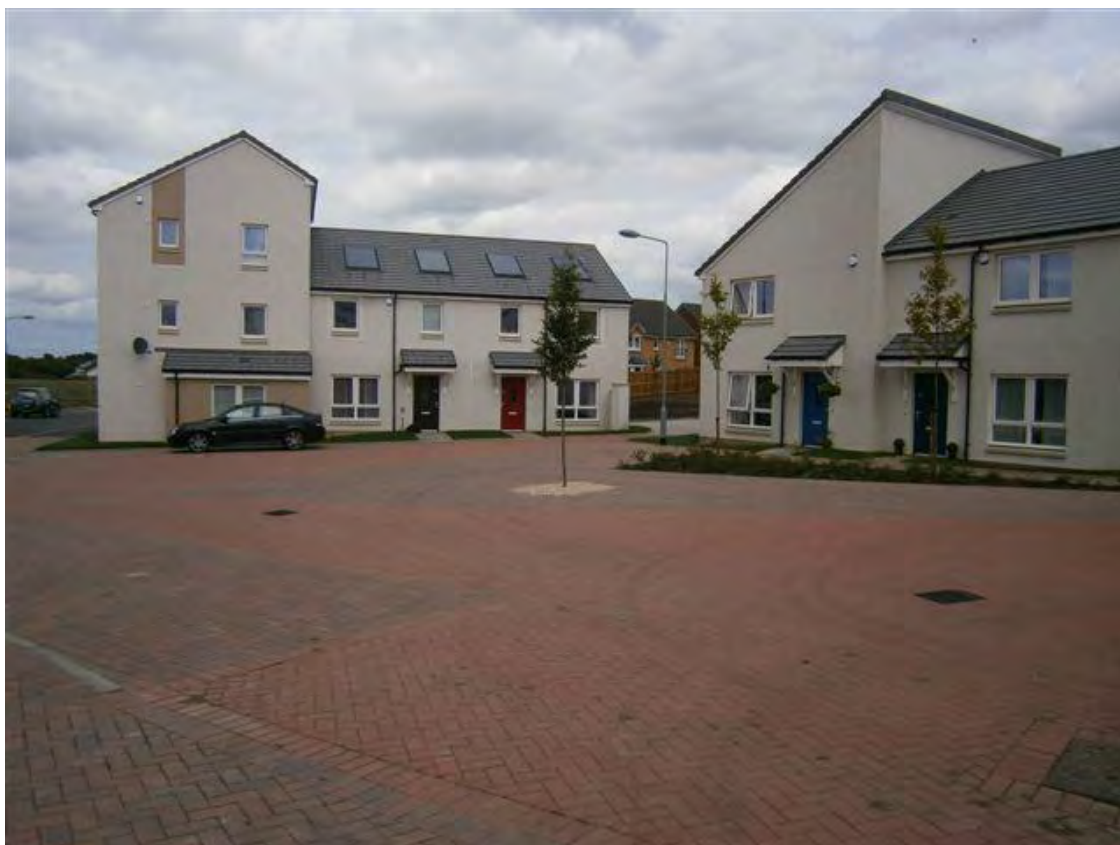
Picture 7 – Fosterton Crescent, Kirkcaldy (better contrast would have been provided with use of buff blocks rather than brindle).
