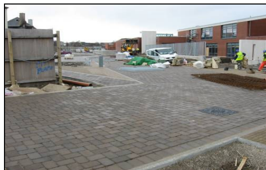
Photo 5. Road Construction Type M2 Completed
