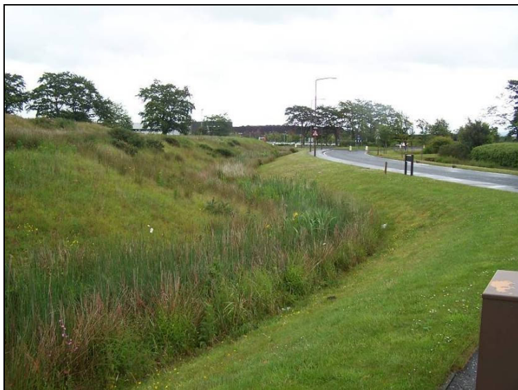
Photo 10. Swale with gully inlets (note kerb and footpath)
