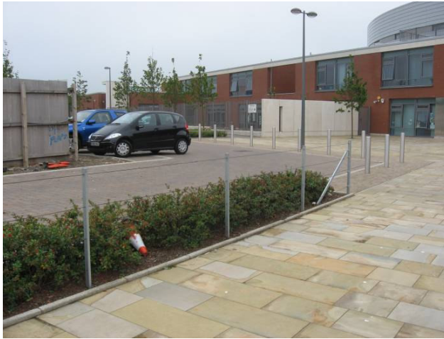
Photo 6. . Different Types of Paving Used on Site.
