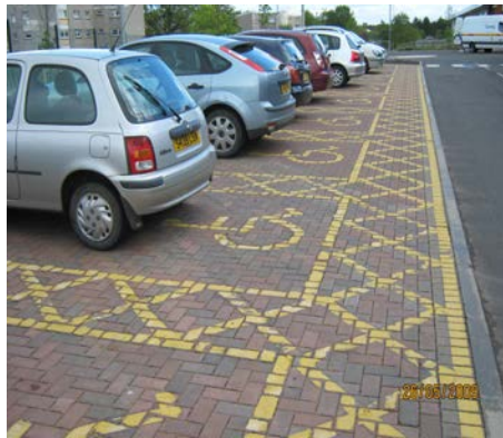
Photo 7. Permeable paving at disabled parking spaces
