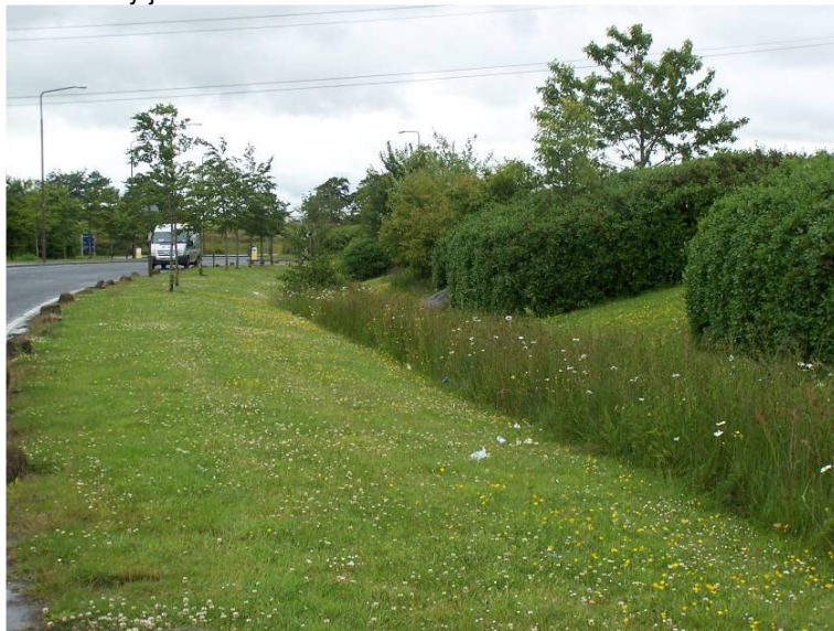
Photo 9. Filter Strip and Swale
