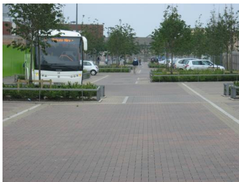
Photo 2. Permeable block paving on the site
