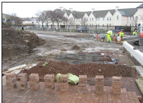
Photo 4. Road Construction Type M1 in Progress
