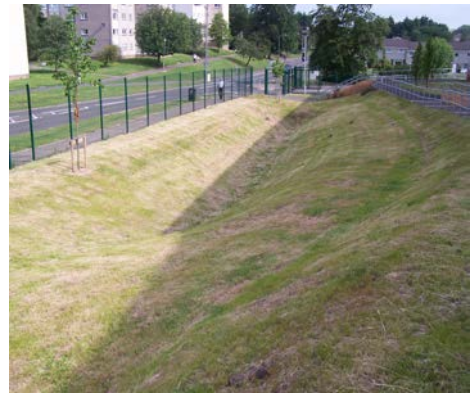
Photo 8. Detention basin with school to right and public road to left
