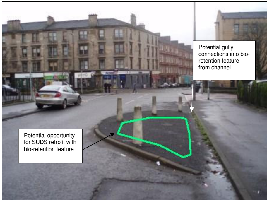
Figure 5.2 SUDS Retrofit in Road Build-out, Glasgow
