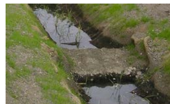
Check Dam to control flow velocity
